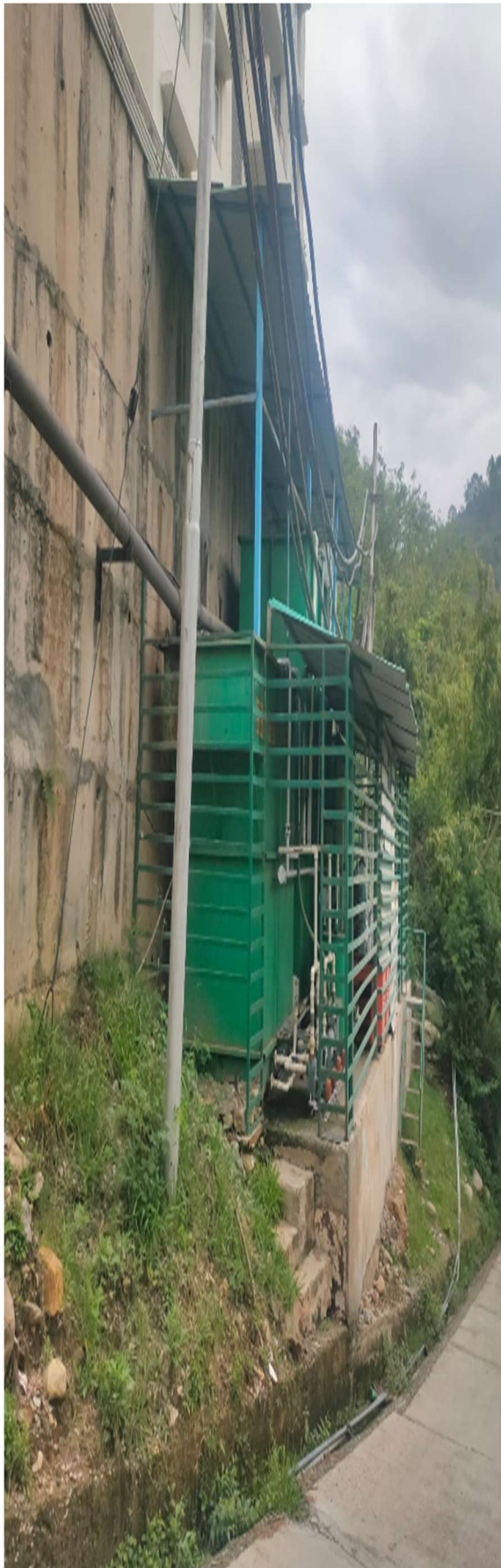
Fig 3: STP Plant (Based on SBR technology) 25 KLD at IIT Mandi
