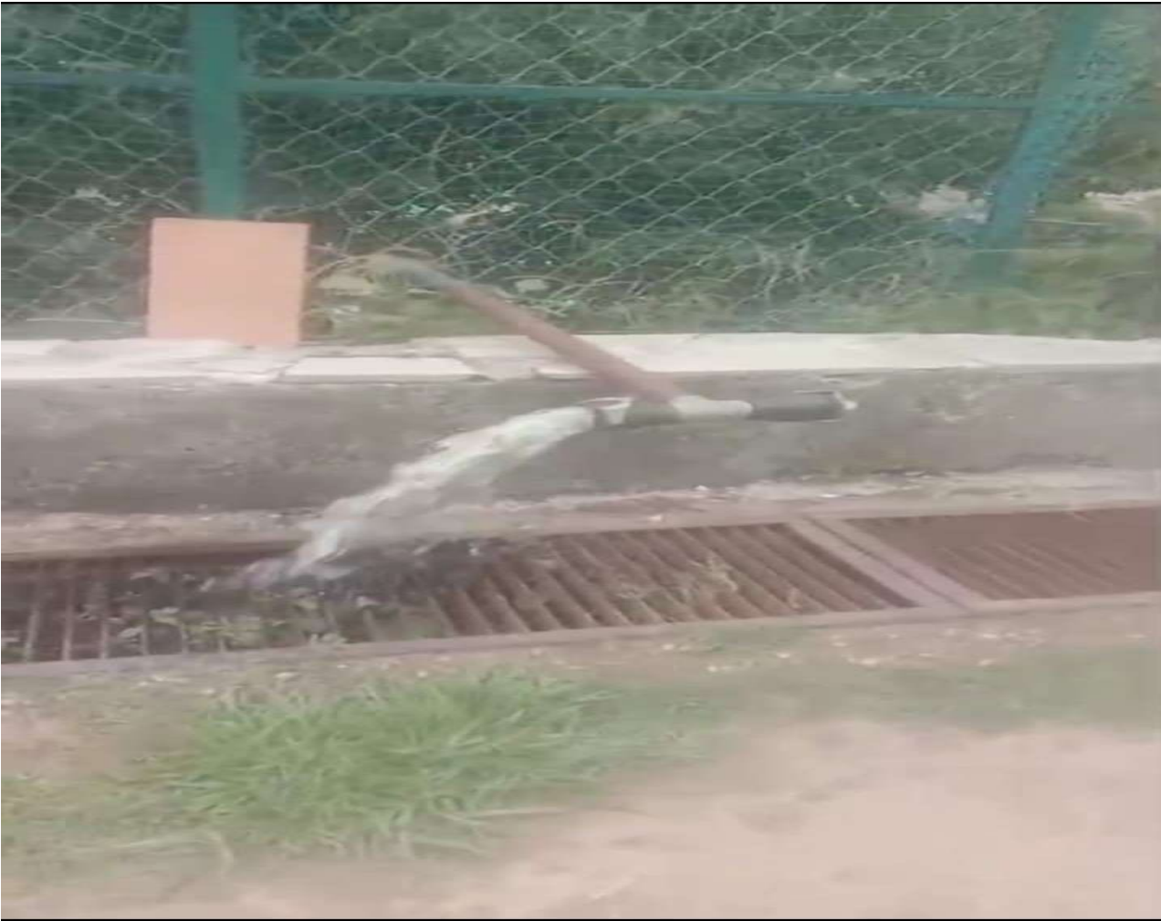
Fig 5: Recycled water for Sports Ground
