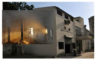
The Fire Safety and Research Laboratory has been developed in collaboration with BARC, Mumbai through the sponsored project of 400 Lac outlay. The laboratory consists of fire test facility for defining the design fire environment relevant for Nuclear Power Plants and other establishments. The main features of the facility are the preparation of actual fire temperaturetime, fire flux- time curves for actual combustibles liquid (cable.
